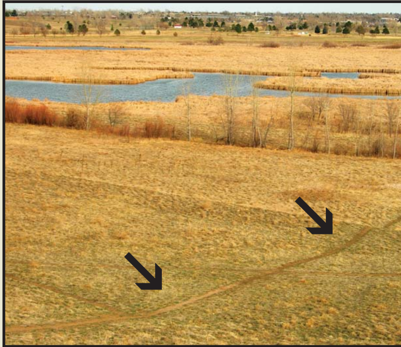
Footpaths like these create erosion and eventually weaken the sides of the dam
